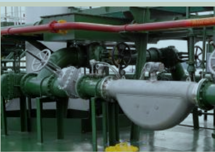
LEGAL DEFENCE: Mass flow meters make it impossible to blend fuels onboard bunker tankers Photo: Sinanju Tankers Holdings
